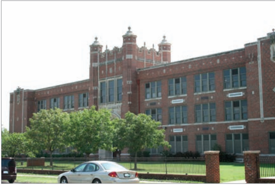
CAPITOL HILL HIGH SCHOOL 500 SW 36TH ST. OKLAHOMA CITY, OK 73109 587-9000
